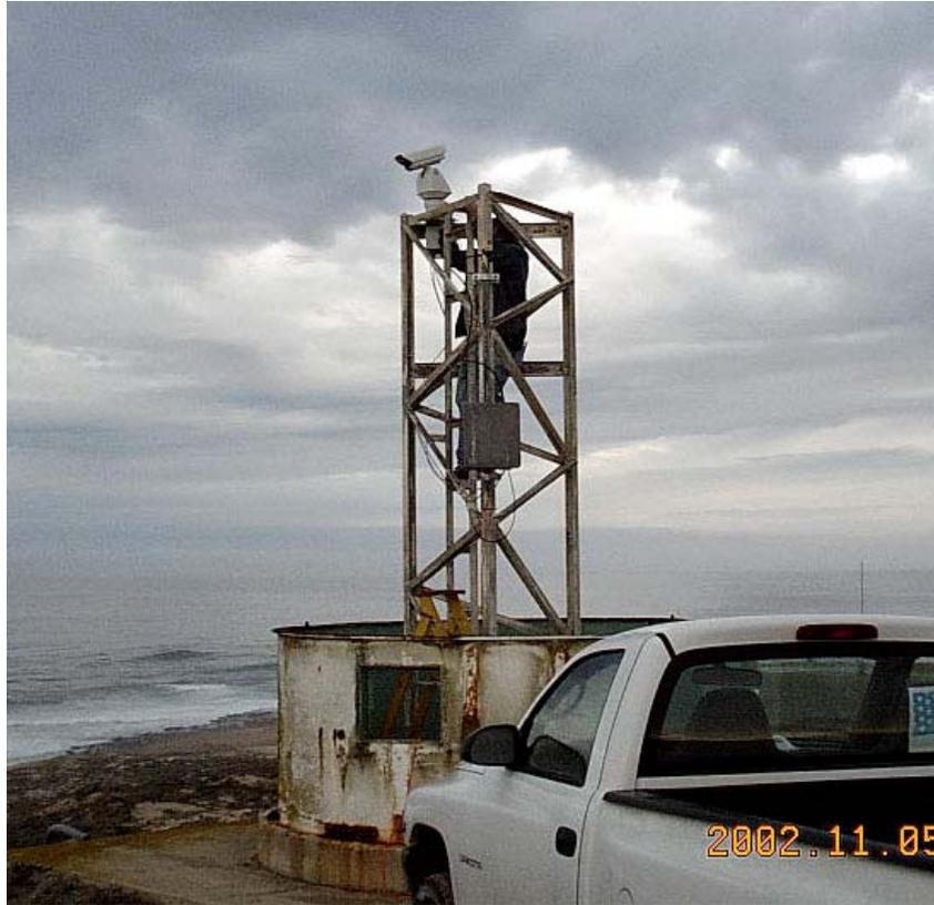
FIGURE 3.2 View of the permanent fixed video camera at Building 809. This camera can be remotely zoomed, tilted, and panned. (Photograph by U.S. Navy)
